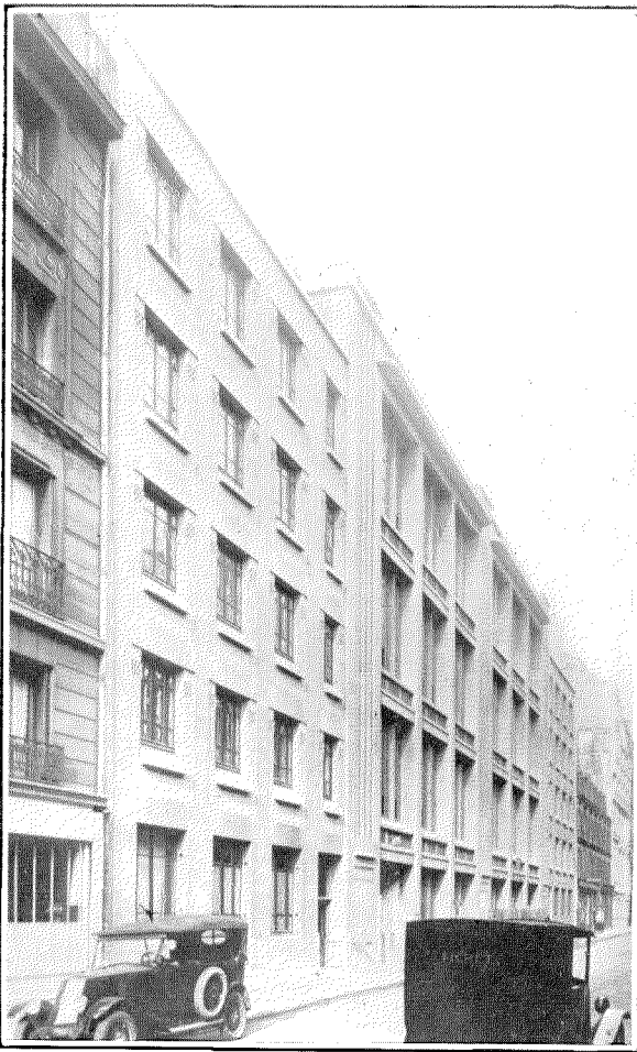
View of the Telephone Building. The wing which contains the new Carnot Exchange is at the rear of the building and runs parallel with the street.
